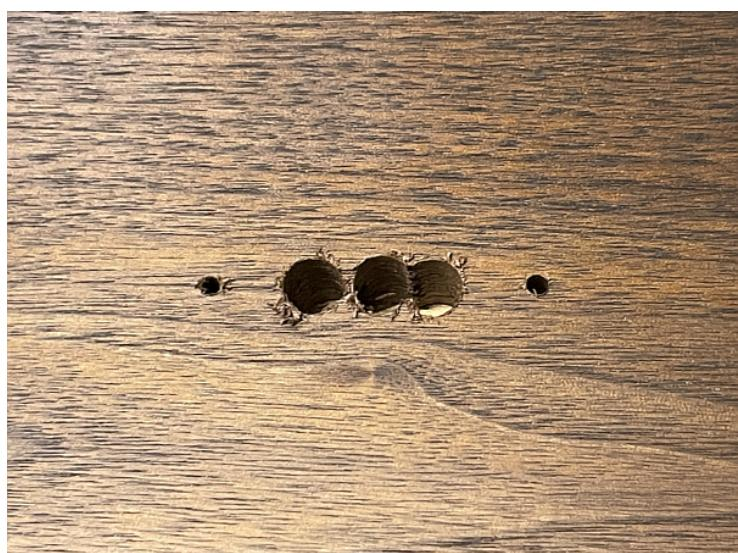
Enlarge the center holes by drilling at an angle in both directions to clear out the wood between the holes. Finish by moving the running drill bit back and forth.
