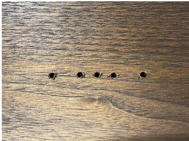
Drill a 5/16" hole in the three center holes. This will be for passing the OLED display through the panel.
