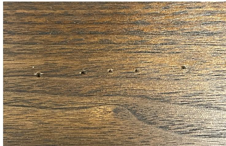
Enlarge the 1/16" holes with a 7/32" drill. This will be the correct size for the bezel mounting screws.
